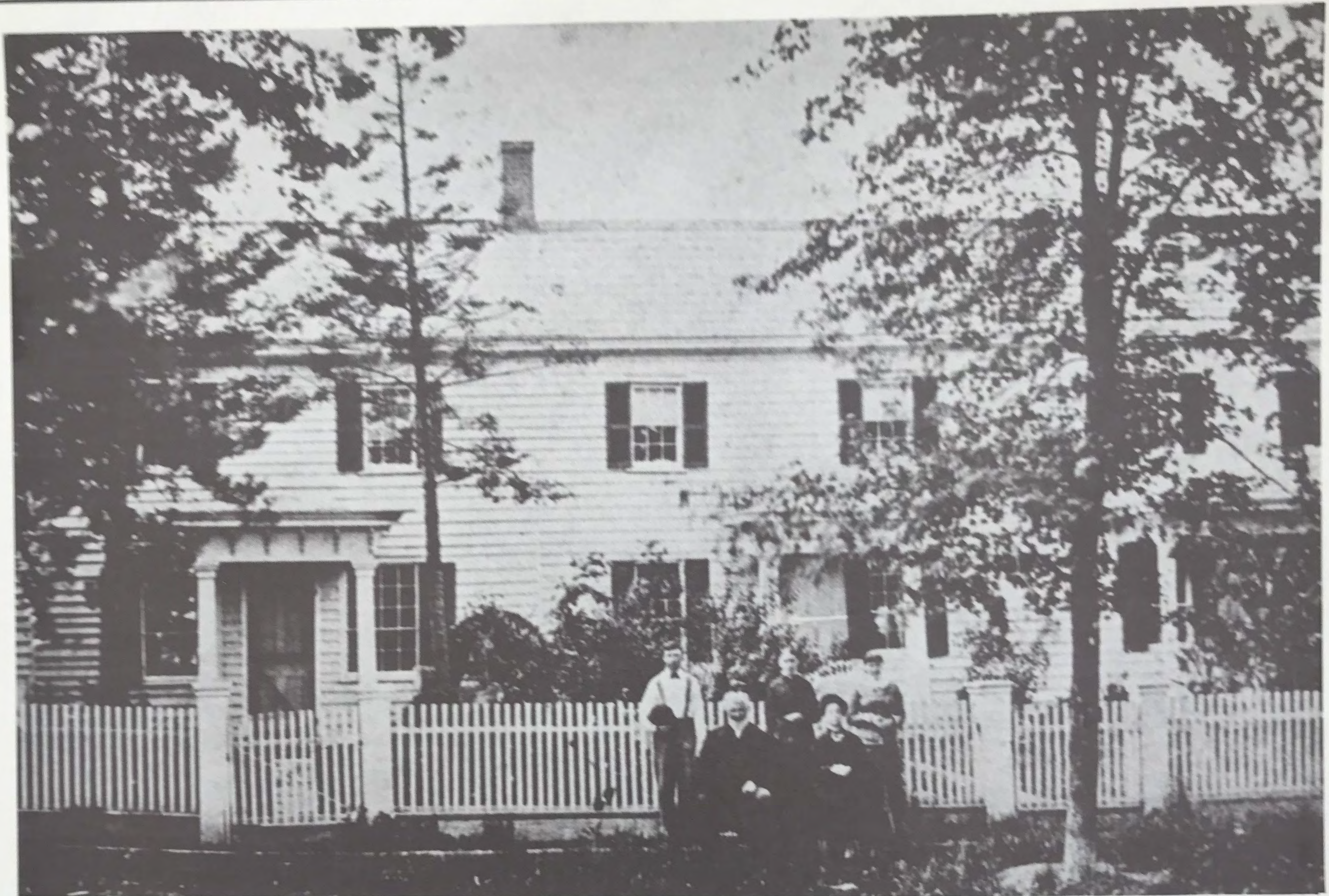
The David Blackwell Family lived and operated a General Store here as early as 1820. Located at 42 East Broad in Hopewell this structure, one of the oldest in town was destroyed in 1987.
