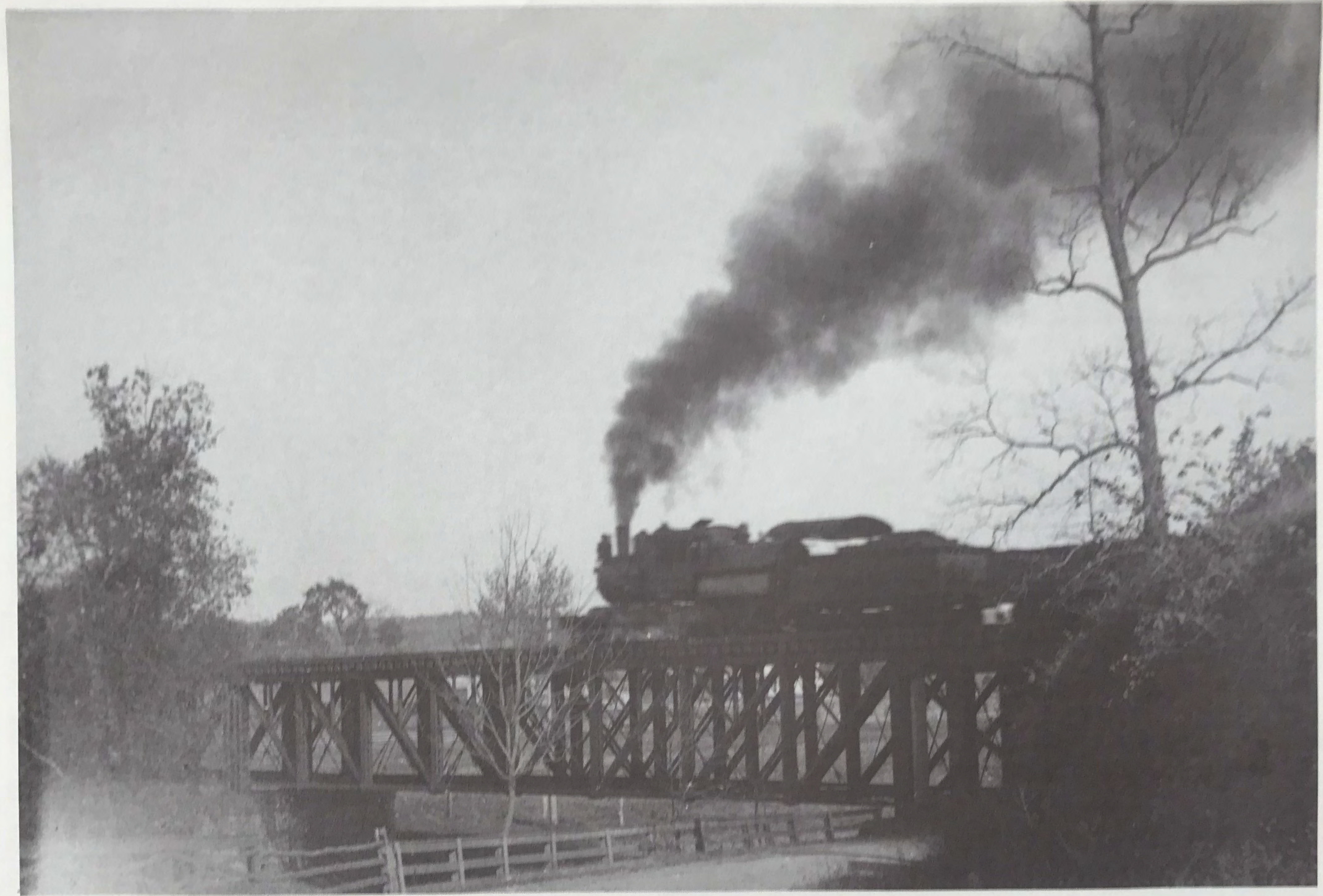
A steam locomotive on the Glenmore bridge east of Marshall's Corner. Built in 1875, the Delaware and Boundbrook Railroad intersected the stock farm of Joseph Moore, now the Hopewell Valley Golf Course.
