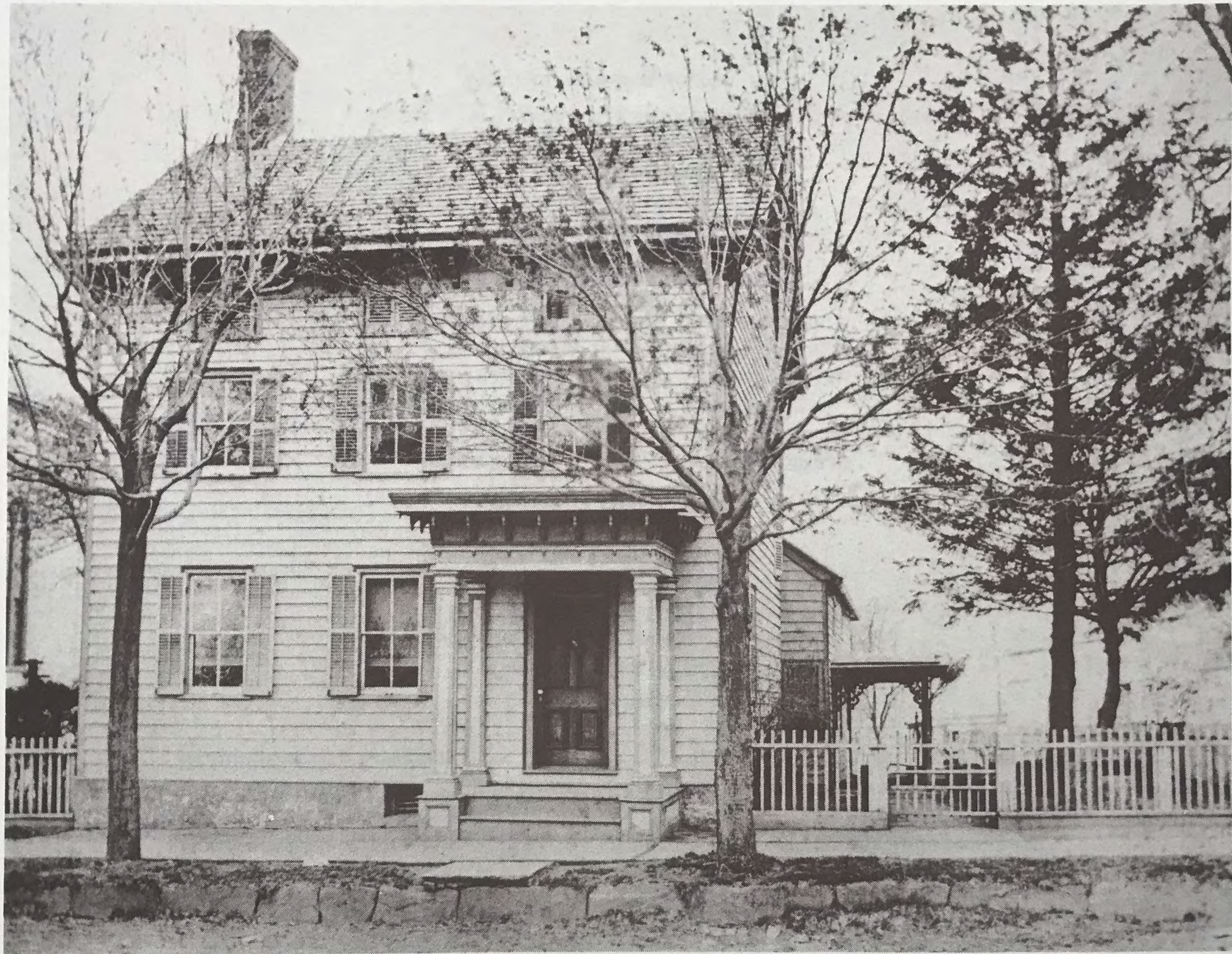
Built around 1820 this house was for many years the home of the Joseph Bunn family. Located just north of the Methodist Church it was from here that Joseph Bunn founded the Methodist congregation in Pennington.
