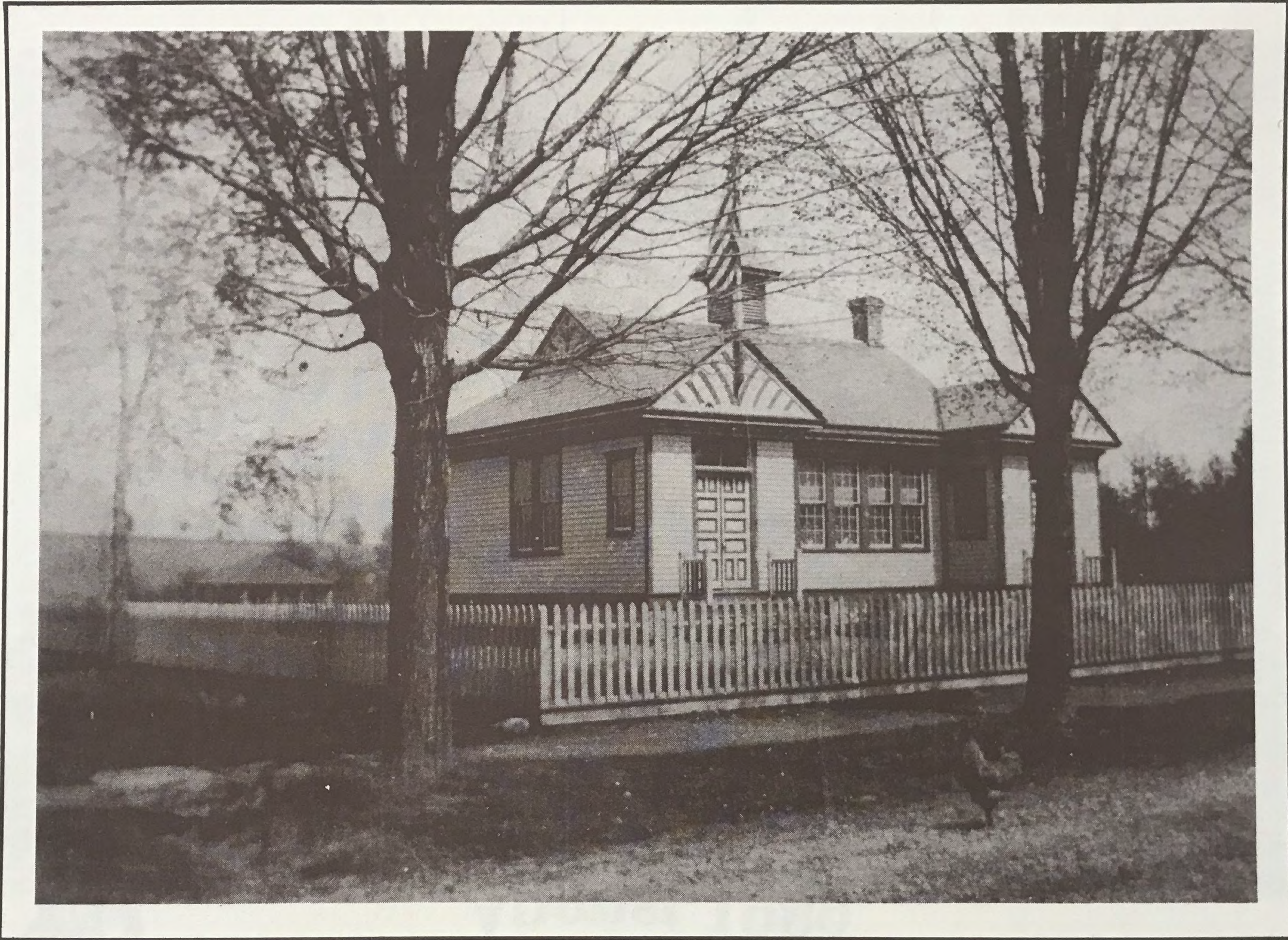
This 1905 photo shows the Titusville School as it originally appeared.
