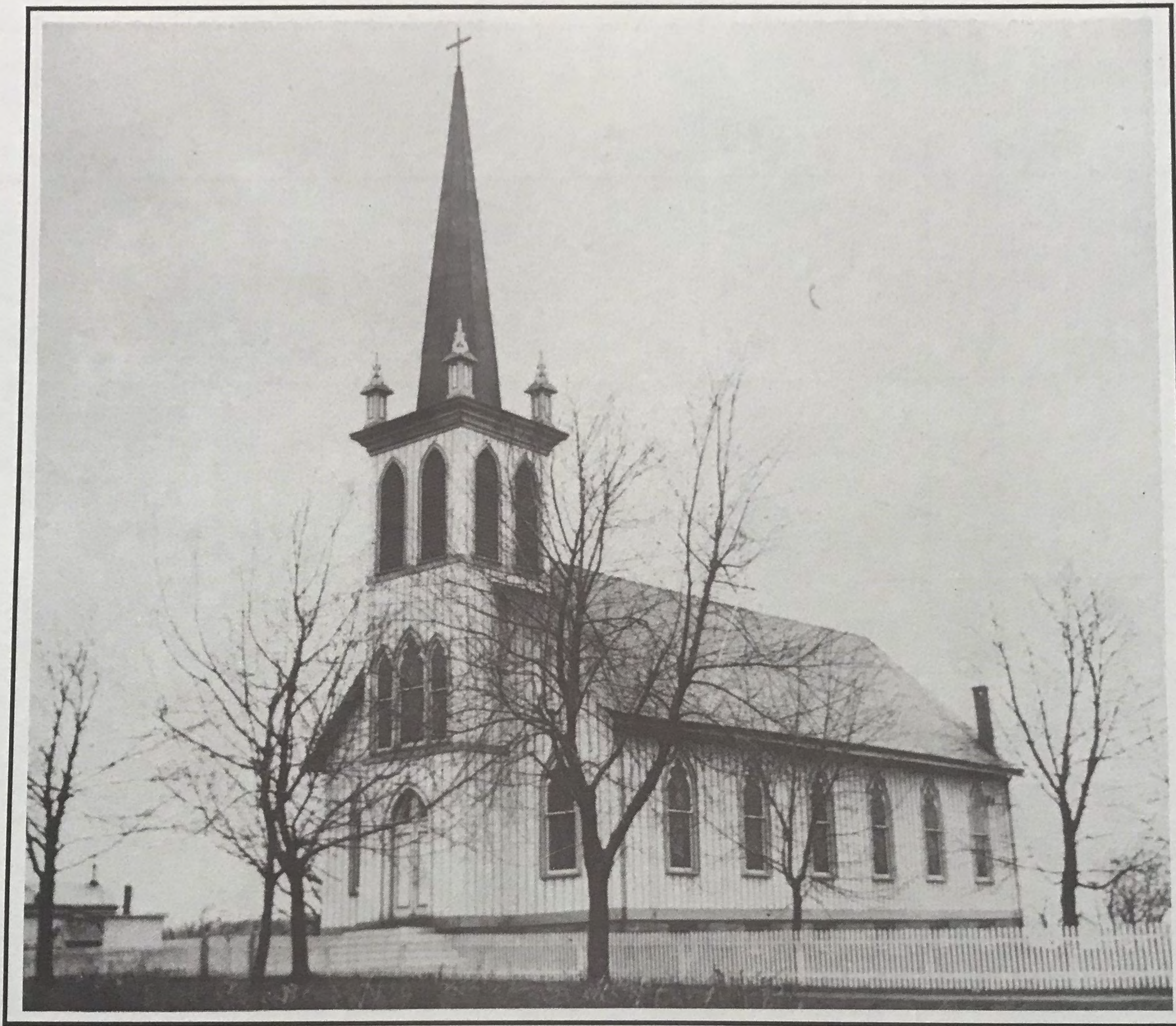
Pictured is St. Alphonsus Roman Catholic Church on Princeton Avenue. Completed in 1878, the structure originally had finials around its steeple and vertical siding.
