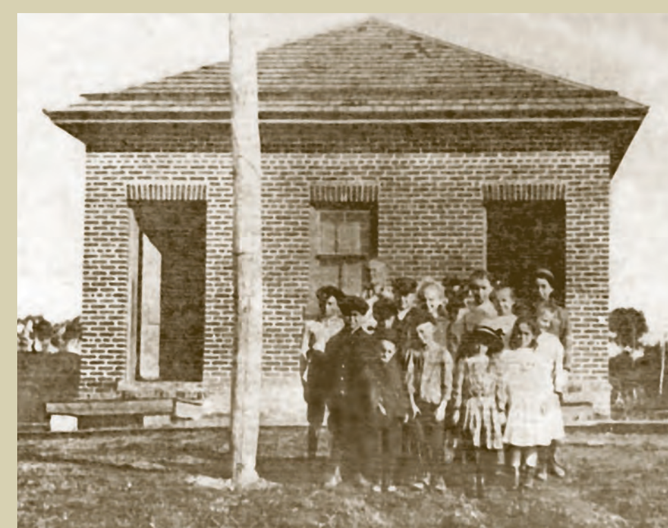
A class photograph, circa 1910, shows the schoolhouse with its original pair of front doors before these were enclosed with a porch and then replaced by a single large door with transom and sidelights [Hopewell Valley Historical Society]
