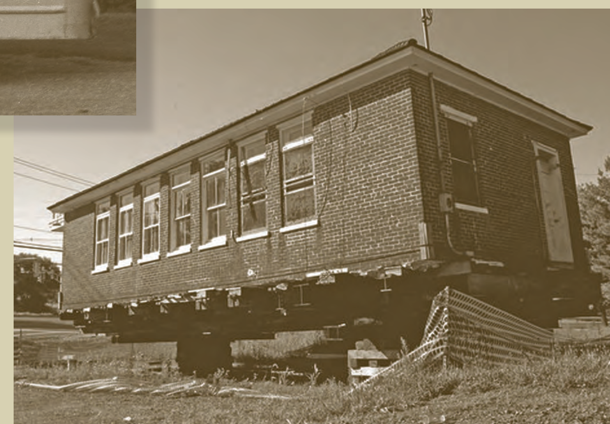
RIGHT: The Hart's Corner Schoolhouse in the process of being moved in 2000 [Hopewell Township Historic Preservation Commission]
