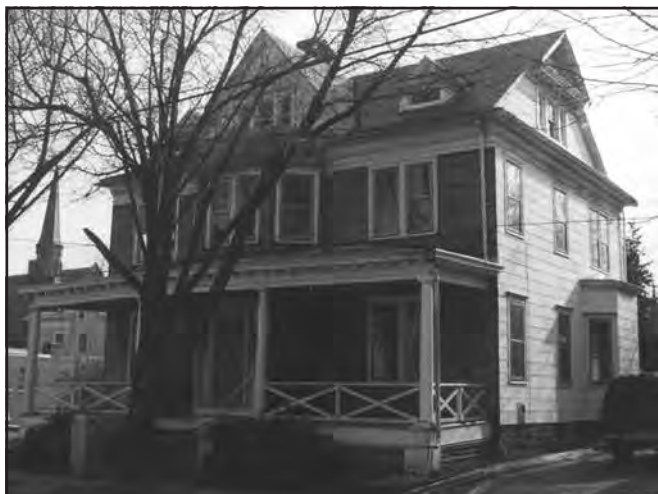
12 West Delaware Avenue in 1999 just as its "restoration" was beginning. Photo by RICHARD BUTTERFOSS
