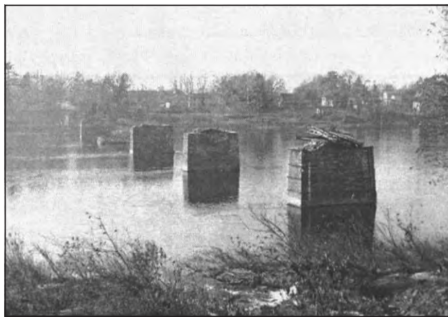
Bridge abutments and remains of the Washington Crossing bridge after the 1903 flood.
