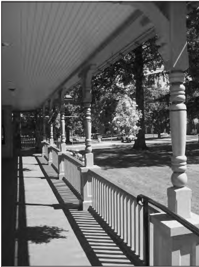
Newly reconstructed wraparound porch.
