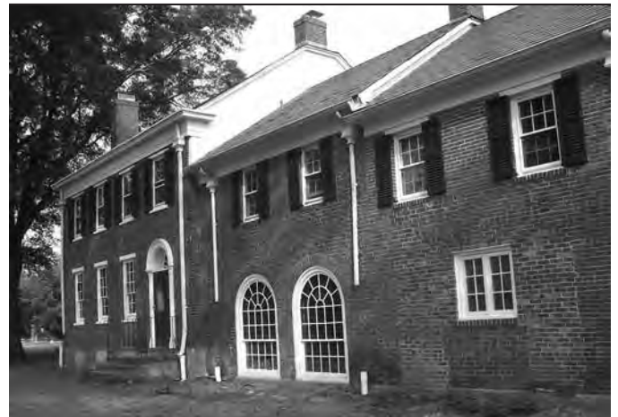
Original Stout-Chorley House and later additions. Photo by Tom Ogren
