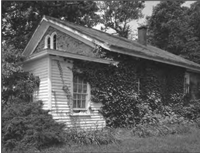
Marshall's Corner Schoolhouse—before restoration (2012)
