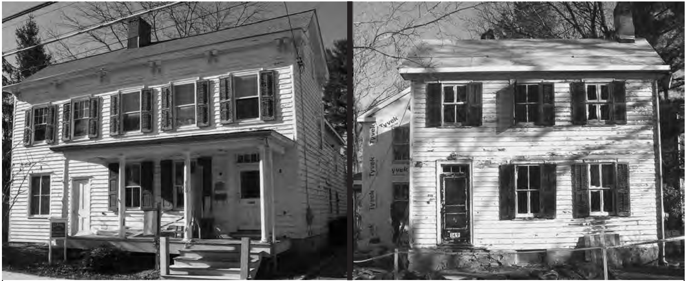
126 (left) and 149 (right) South Main Street, both circa 1840, before restoration.
